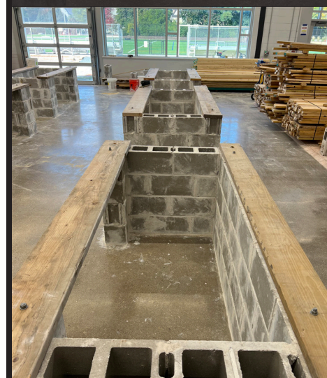
Photo of the bathroom build that students construct from bottom to top.
