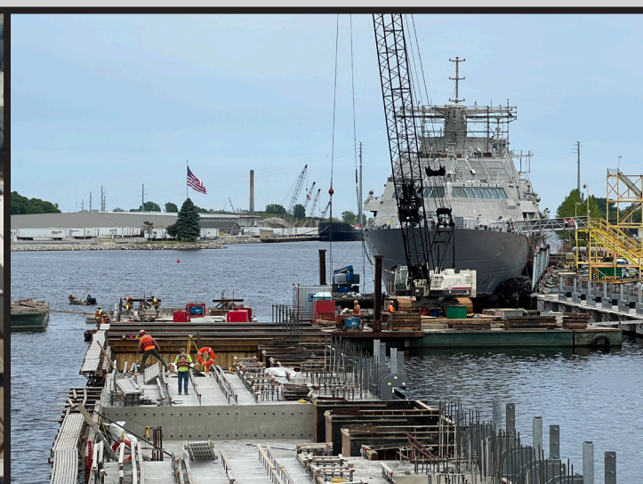
Photo of Fincantieri's shiplift under construction.
