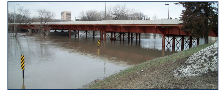
1st Avenue North bridge in Moorhead, MN was impassable due to rising Red River waters in 1997.
