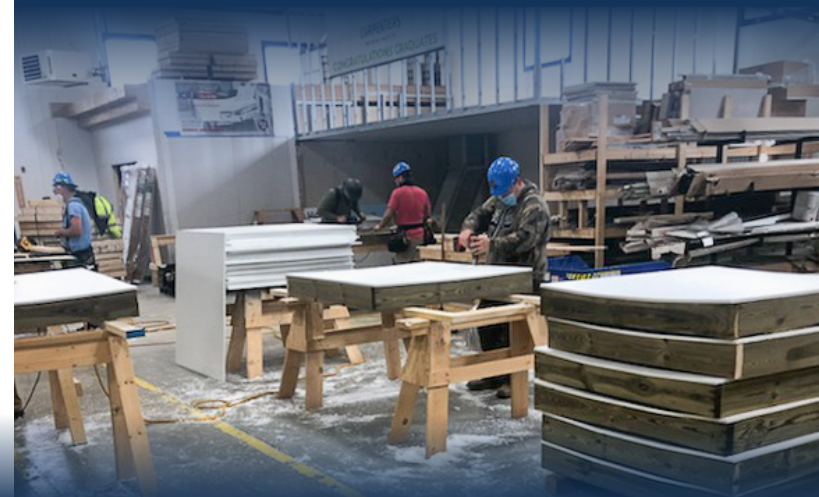
Duluth apprentices construct new hockey rink walls in the Hermantown Training Center.
