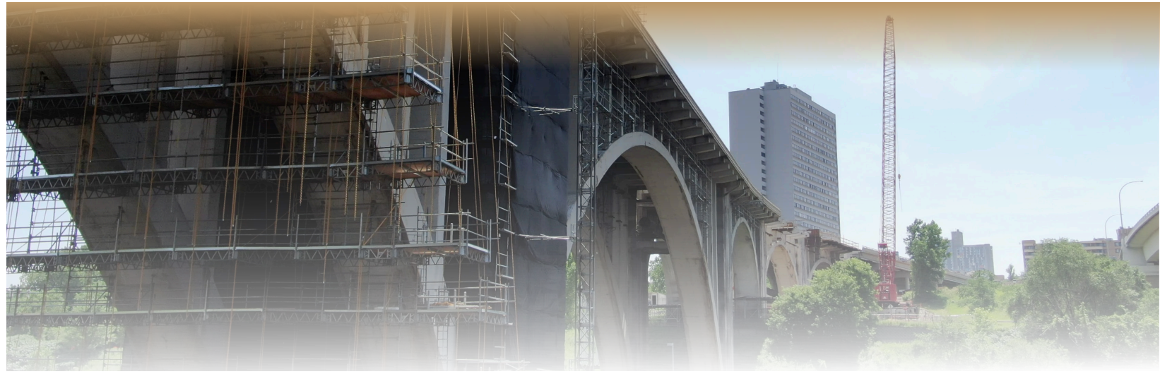
Minneapolis Tenth Avenue/Cedar Avenue bridge repairs.
