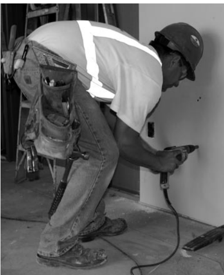
NPD, Inc., foreman Al Kroll, Local 68
