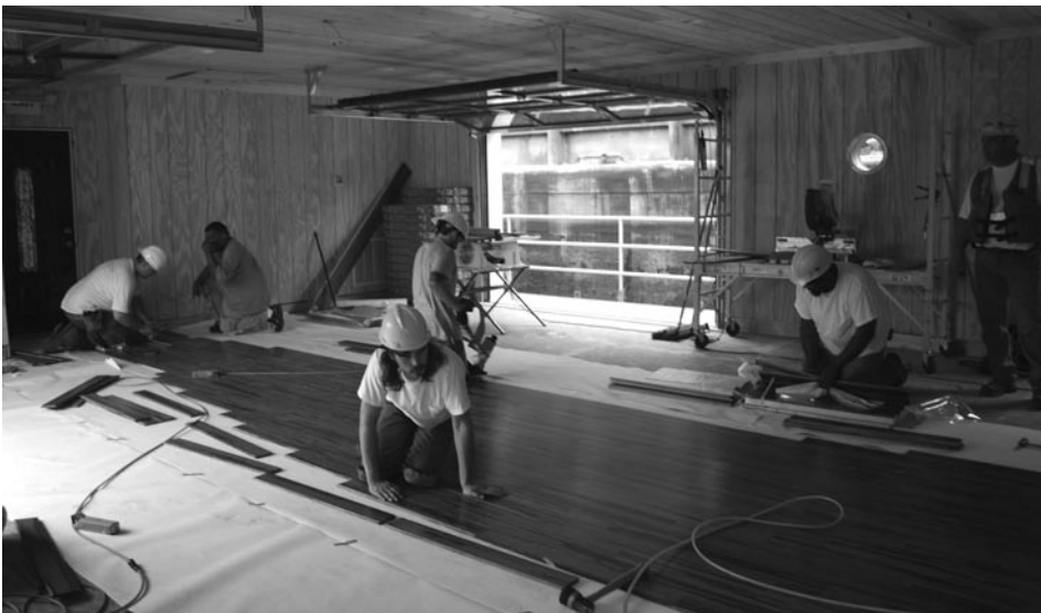
Floor covering apprentices install solid bamboo flooring in the barge classrooms.
