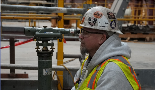
Todd Korpela (Local 1348 - Virginia, MN) precision leveling a sole plate
