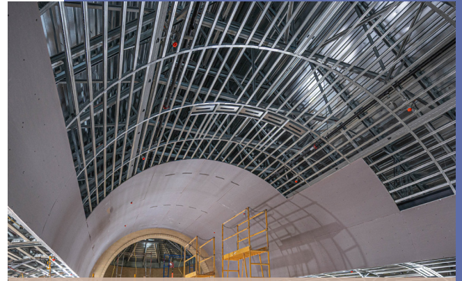
Photo of the Armstrong Grid ceiling system in the chapel.
