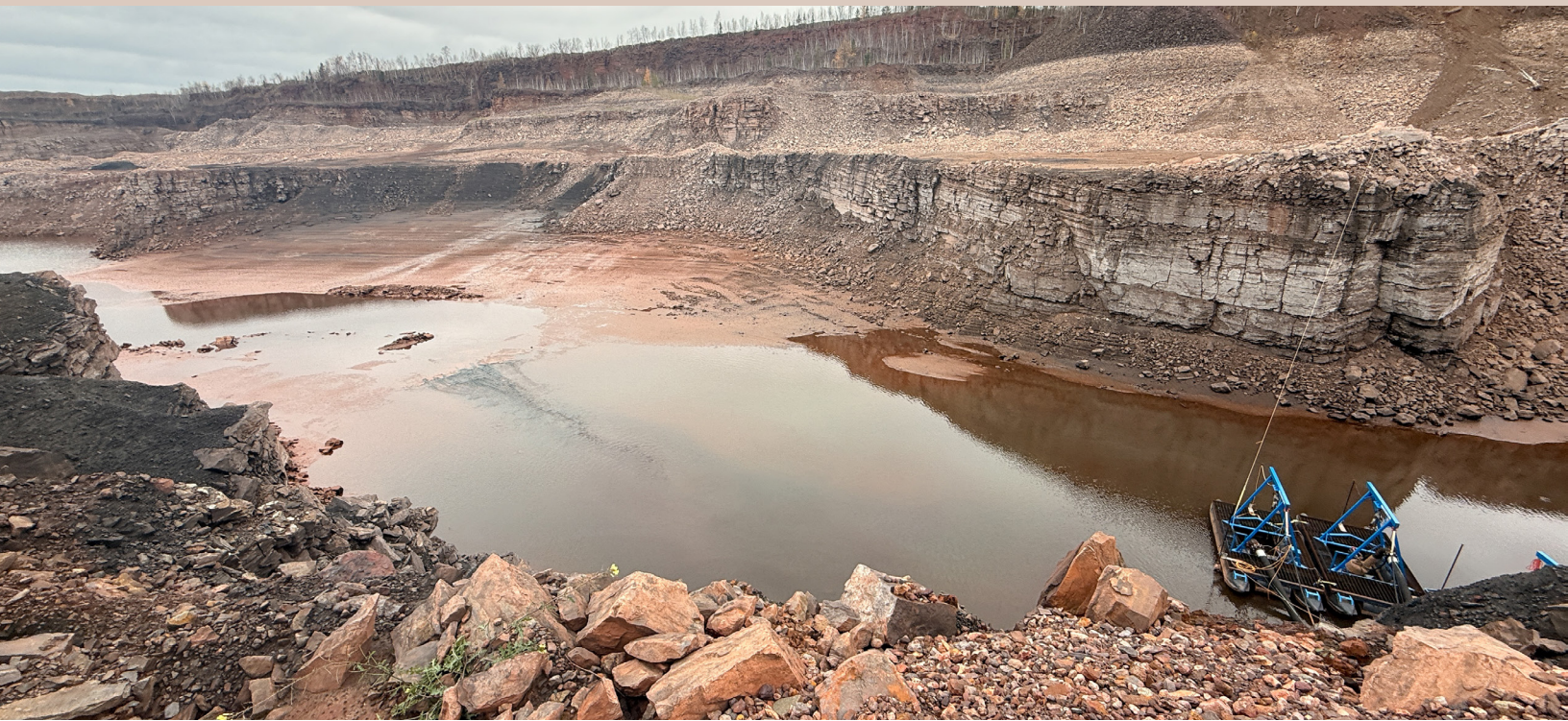
Pit 5, which is 5/8 of a mile from the facility, was dewatered starting in April 2024. At the time, it held 4.5 billion gallons of water. Seven pumps removed 15,000 gallons of water per minute. In August 2025, the pit was down to 750 million gallons. This photo was taken on October 28, 2025.
