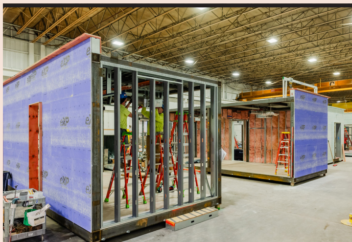
Crew assembling a modular unit at Boldt's prefabrication facility in Oshkosh, Wisconsin.
