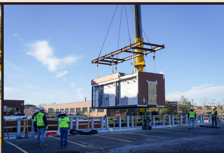
A modular unit being transported for on-site installation.
