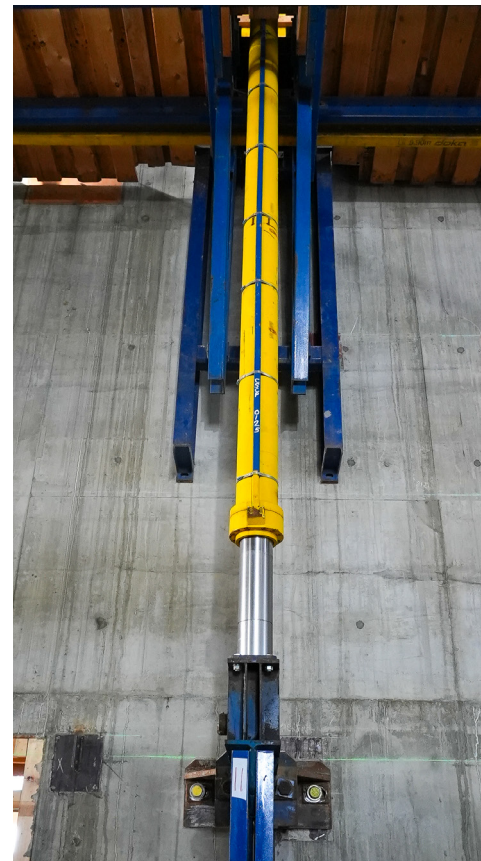
One of the eighteen DOKA Shear Core Climber hydraulic cylinders.
