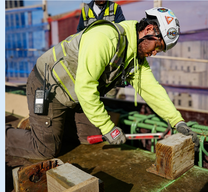
Diego Kyndt (Local 427 - Omaha, NE) installing edge form.
